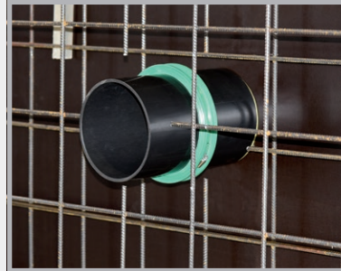
DURO Plus in bekisting
